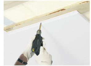
Focus F installeras genom skruvmontering
